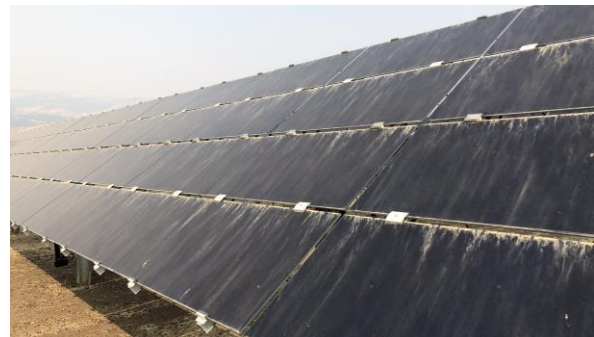
Dust and dirt on a solar array at California Flats before panel cleaning
