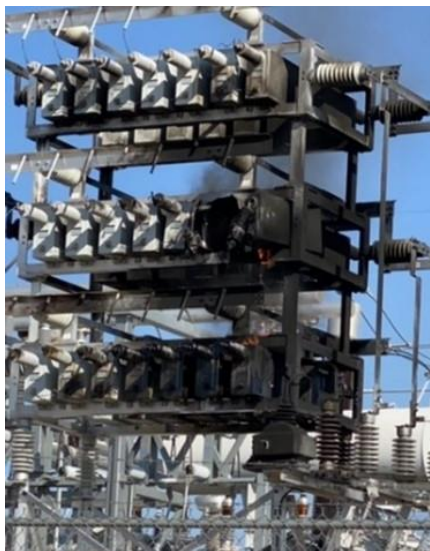
Example of an ESG notification due to a fire in capacitor bank at Moapa Southern substation
